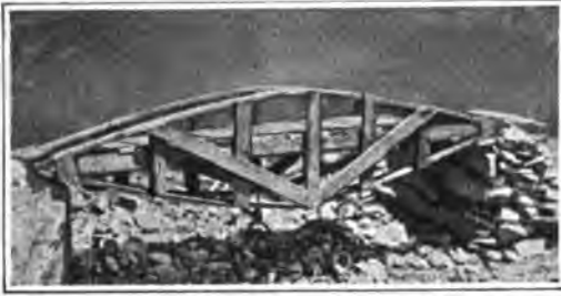
PRELIMINARY 3-FOOT MODEL OF THE BOWSTRING SPAN
